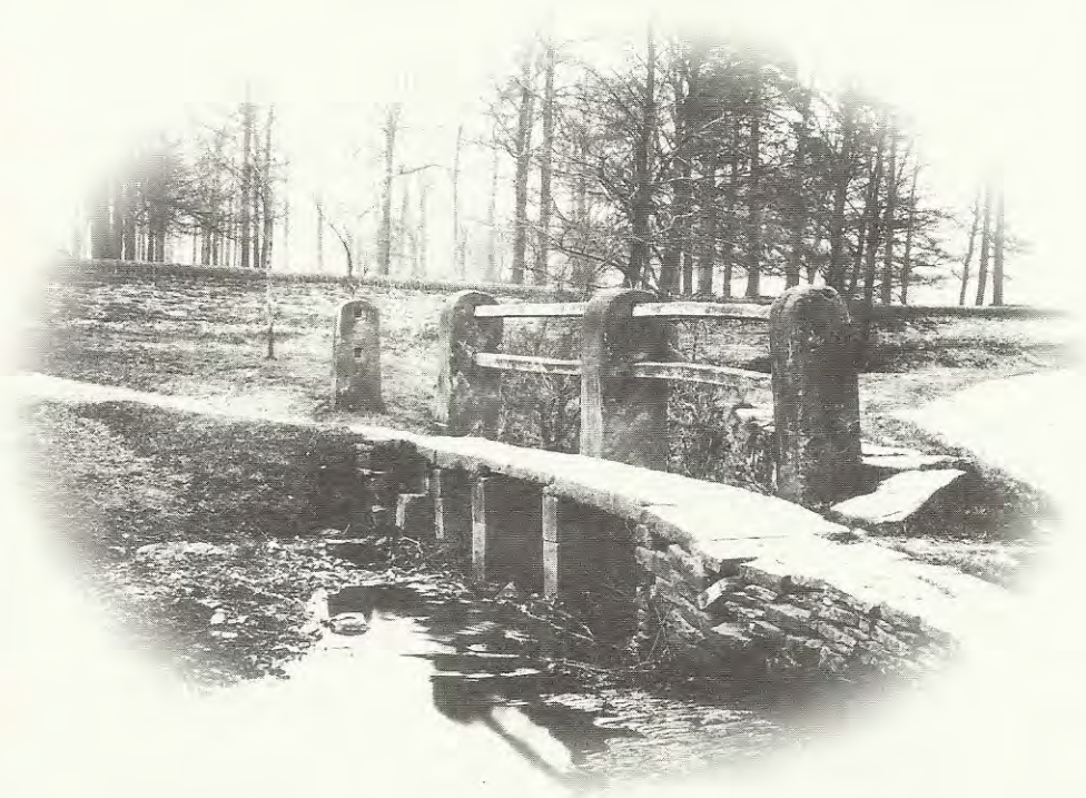
Clapper Bridge c. 1904 at junction of Bridleway Nos 1 & 6
