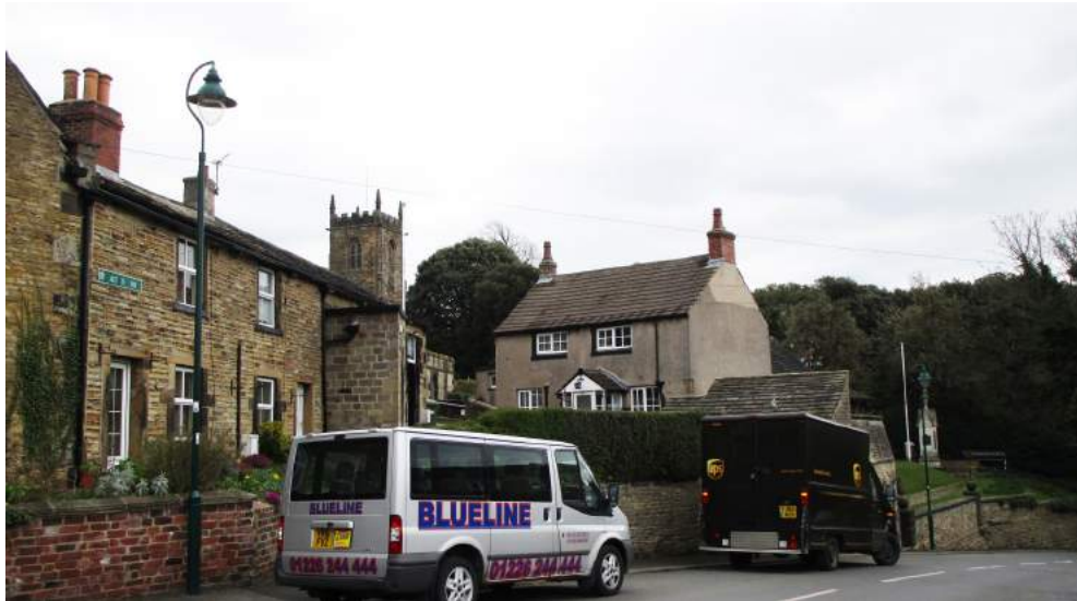
Plate 9: View of church tower, Hill Top
