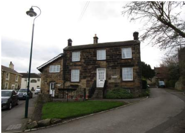
Plates 49 and 50: UPVC doors and windows replace historic features and undermine the character and appearance of the conservation area
