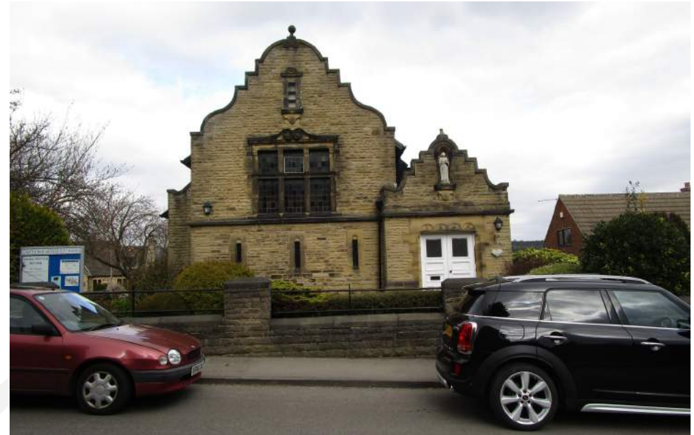
Plate 10: Cawthorne Methodist Church, Darton Road
