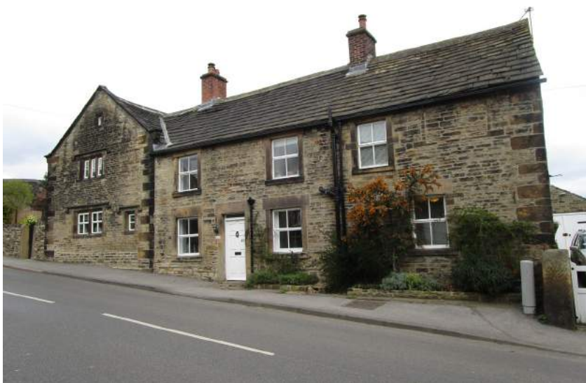
Plate 35: Nos. 31 and 33 Darton Road
