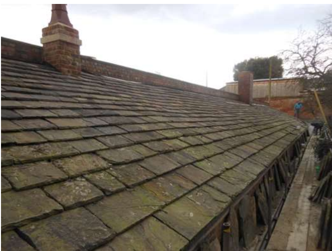
New roof on the North Range almost complete.
