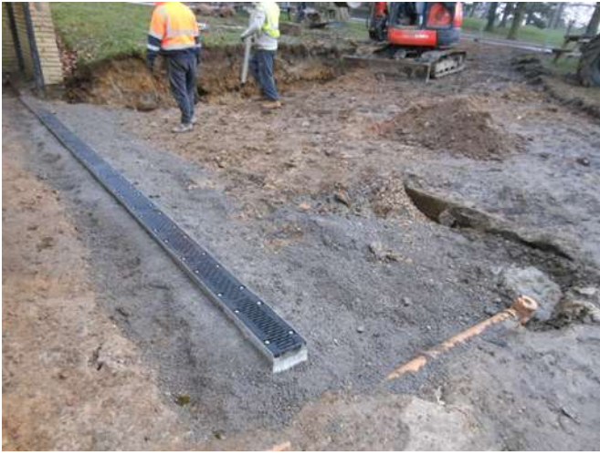
New drainage and retaining wall being installed by the Pavilion to make a nicer welcome and more space.
