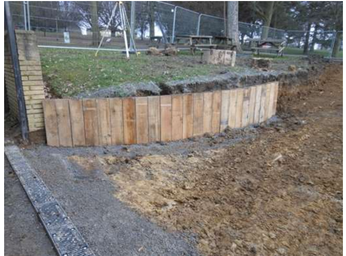
New drainage and retaining wall being installed by the Pavilion to make a nicer welcome and more space.
