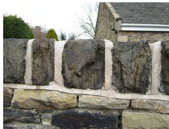
Plate 51: Ribbon and cement pointing detract from historic walling and is a cause of erosion
